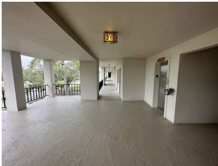
Figure 6: Walkway and Terrace, Level 4
